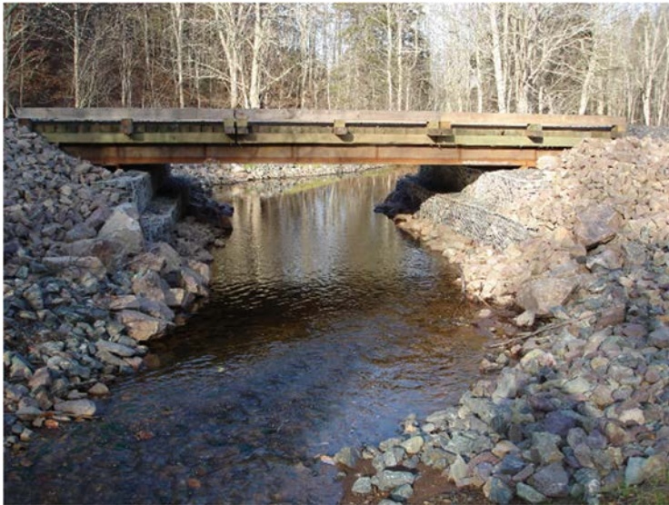
New bridge installation, Paul MacDonald, PHP
